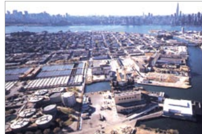
Newtown Creek WPCP on the East River.
