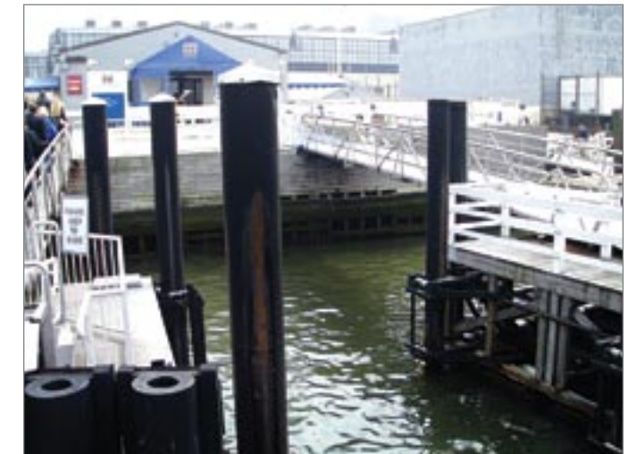
West Midtown Ferry Terminal on the Hudson River. AKRF helped the New York City EDC develop a new terminal to serve New Jersey commuters.
