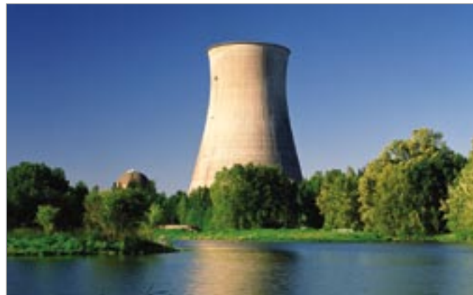
Cooling towers minimize water intake.
